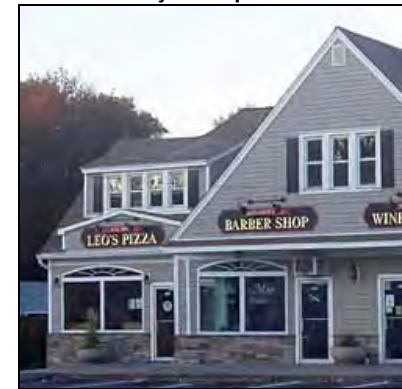
After Façade Improvement
