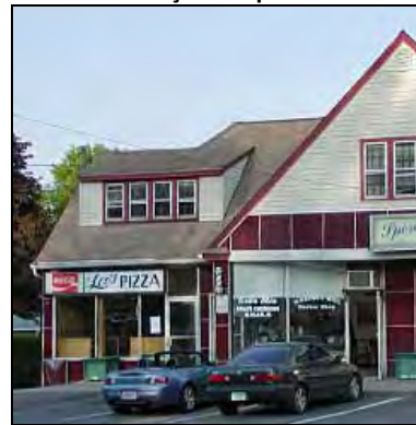
Before Façade Improvement
