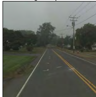
Residential Street With High Utility Value
