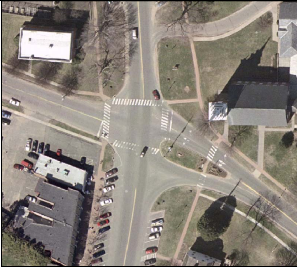
Existing Conditions, Main, Church and Marsh Streets
