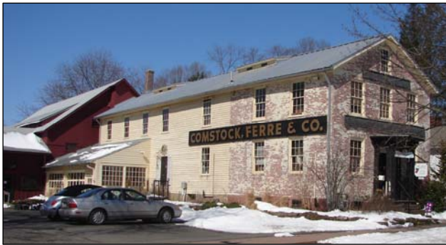
Historic building on the Comstock, Ferre & Co. property
