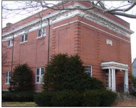
Existing conditions of the Masonic Hall
