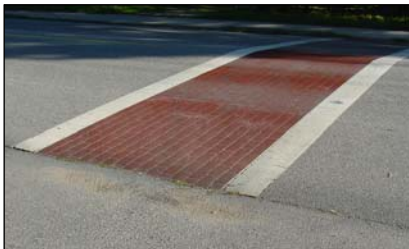
Landscaped medians and material changes at crosswalks help to visually slow traffic
