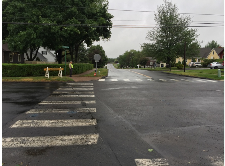
Figure 13: Sample Crosswalk on Route 2
