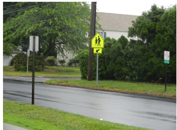
Figure 18: Crosswalk Sign with No Corresponding Crosswalk in Road
