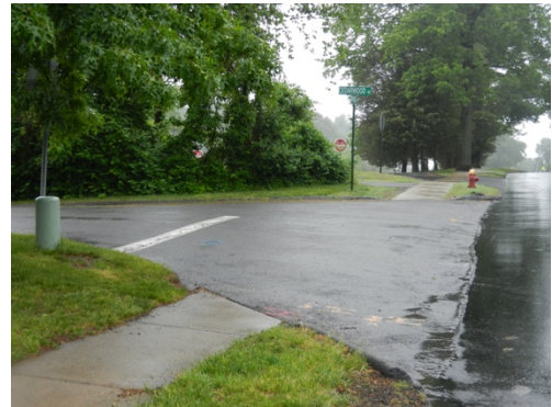
Figure 26: Sidewalk Ramp Lacking ADA Compliance
