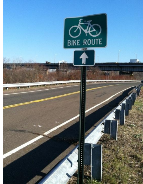
Great Meadow Road in Wethersfield is part of the Heritage Way Bikeway. Putnam Bridge is visible in the background.
