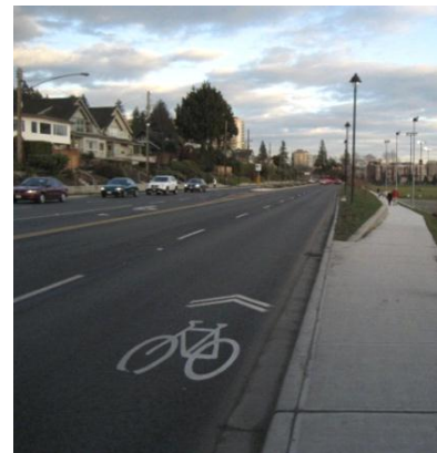
Example "sharrow" marking located along the curb of a shared travel lane.
