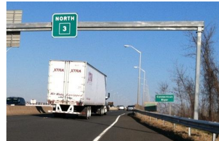
Overhead sign structure at western end of the Putnam Bridge
