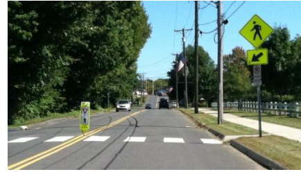
Representative mid-block crosswalk with pedestrian warning signs (Glastonbury)
