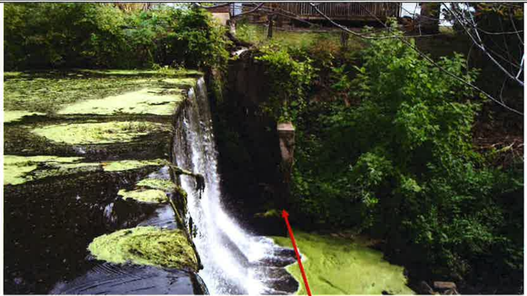
Former turbine housing structure
