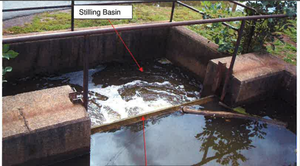
Spillway with Stop Logs
