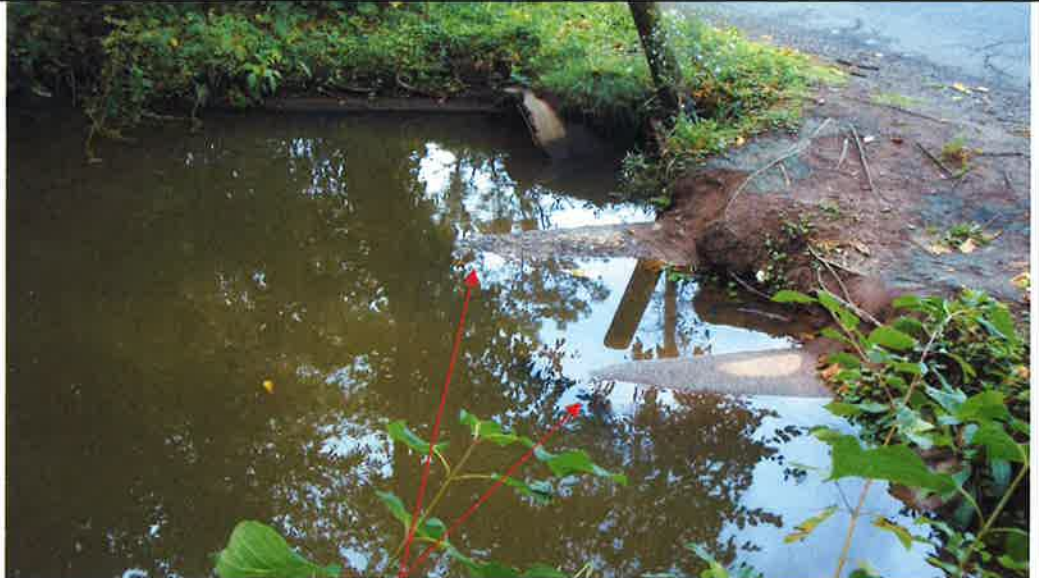
36-inch diameter RCP Pipes
