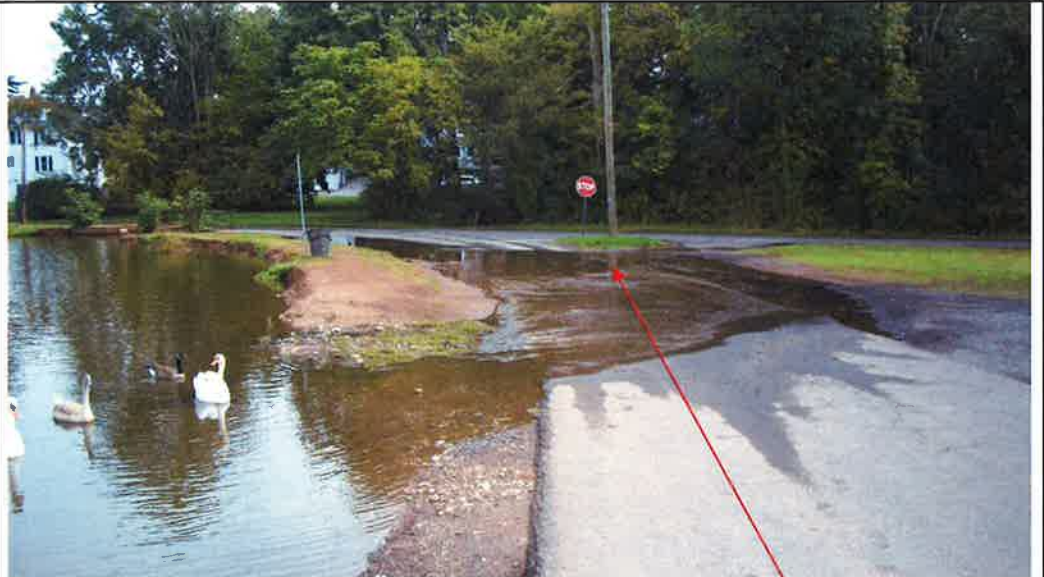
Submerged Stormwater Catch Basin
