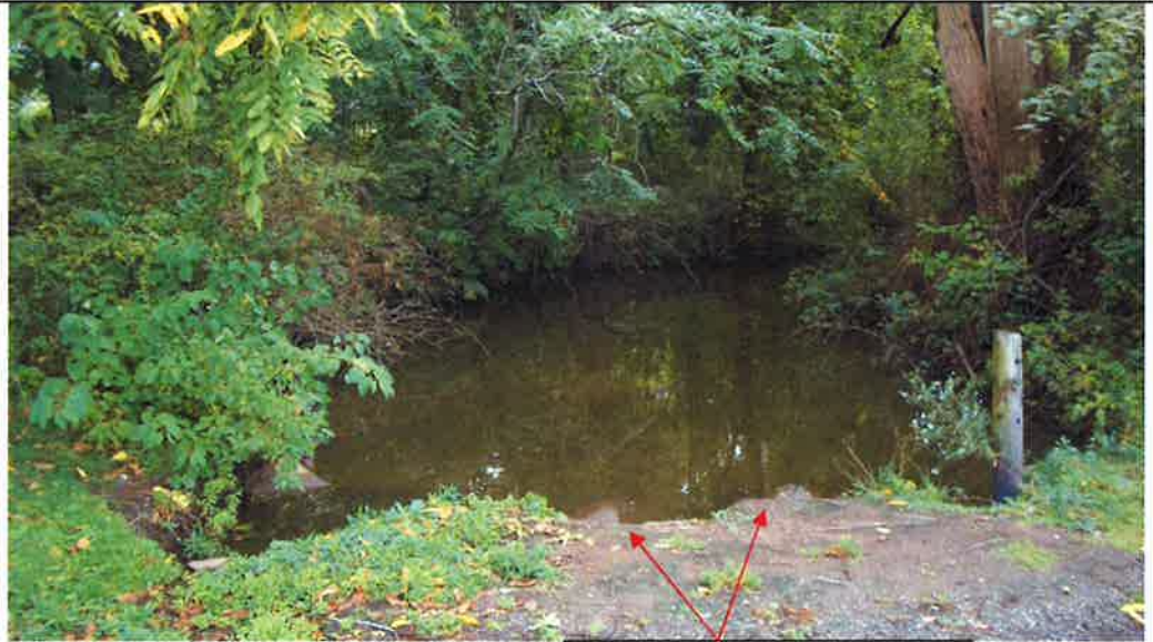
36-inch diameter RCP Pipes
